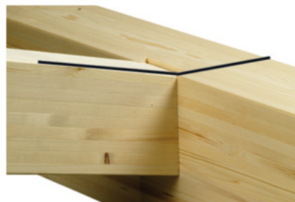
Rafter to base plate (wall beam)
