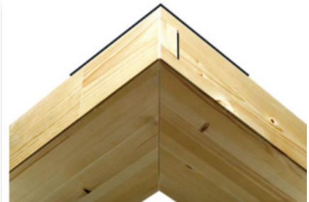
Rafter-to-rafter (without ridge purlin)
