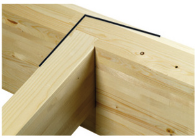
Rafter to chamfered ridge beam
