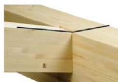
Rafter on head plate
