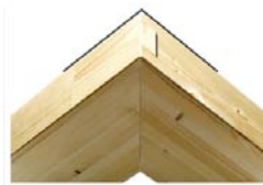
Rafter-to-rafter (without ridge purlin)
