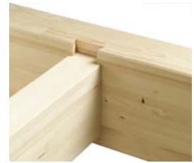
Joist offset from stringer
