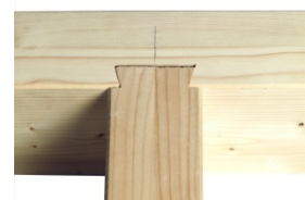
Joist flush with stringer
