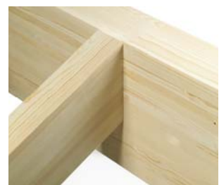
Rafter on squared ridge purlin
