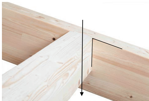
A principal rafter and its purlin fitted together. The rafter is reclined and the purlin is straight.
